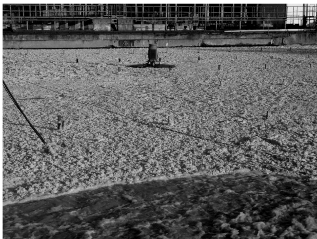
Fig. 1. Foam on the surface of activated sludge in the WWTP of ZPM "Mlekpol" in Mrągowo
